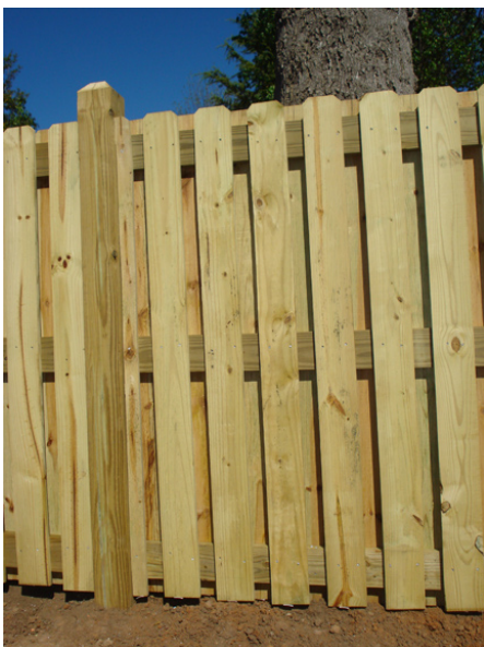
Two-Sided Privacy Fence.
