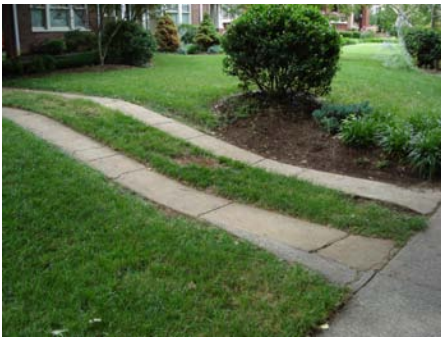
Concrete Parking Strips
