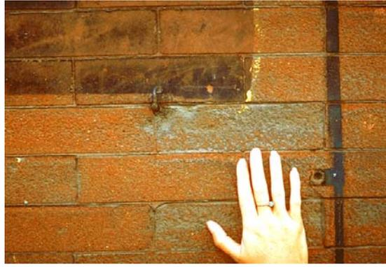
*Sandblasting removed the outer surface of this brickwork, exposing the soft interior to water penetration and subsequent freezing and thawing damage.*
